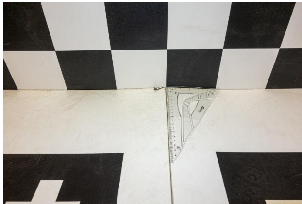
Finding a line perpendicular to the wall
